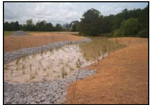
In the second phase of the project, portions of three deep ponds were converted to wetlands (photos above).
