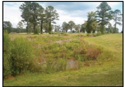
About 15 acres of wetlands were constructed during the first and second phases of the project.
