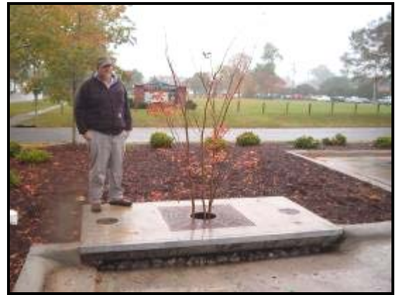
Scott Alons of Chowan Soil and Water stands next to the stormwater filtration system at John A. Holmes High School in Edenton. This is the first system of its kind installed in North Carolina.
