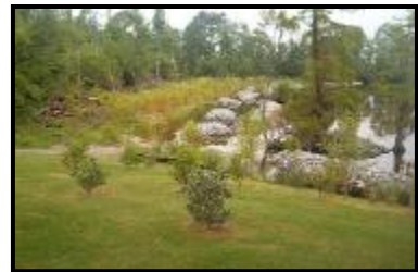
1,000 ft of Stabilized Shoreline
