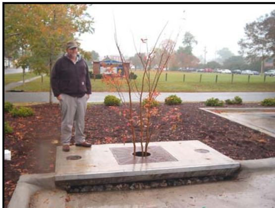
Scott Alons of Chowan Soil and Water stands next to the Filterra® stormwater filtration system at John A. Holmes High School in Edenton. This is the first system of its kind installed in North Carolina.
