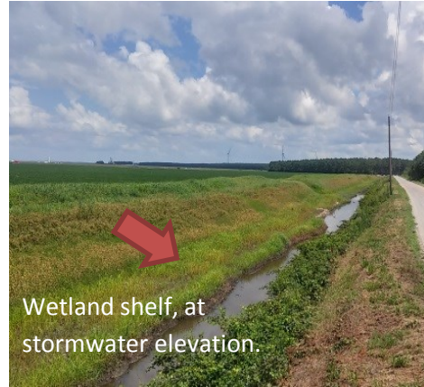
Wetland along 4,800' of main drainage canal with seeded bank and wetland plants along shelf. View looking northeast.
